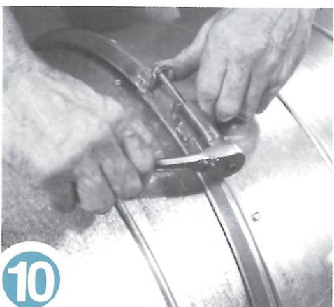
10 Tighten the bolt on the Closure Ring until it makes even contact around the circumference of the duct sections.
