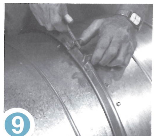
9 Slide Closure Ring over mating Flanges and insert bolt.
