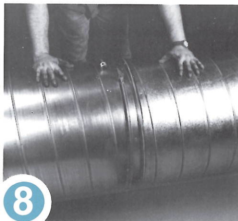
8 Slip outer Closure ring over end of duct. Align Flanges on mating duct sections before they touch.
