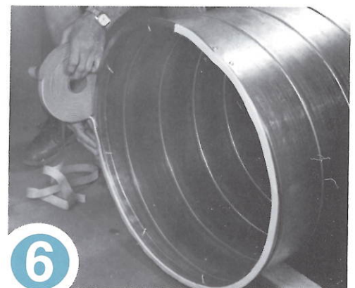
6 Complete the gasket application by installing gasket on the face of the Flange around the entire circumference of one of the mating Flanges.
